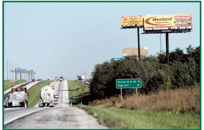
New Billboards on I-70
